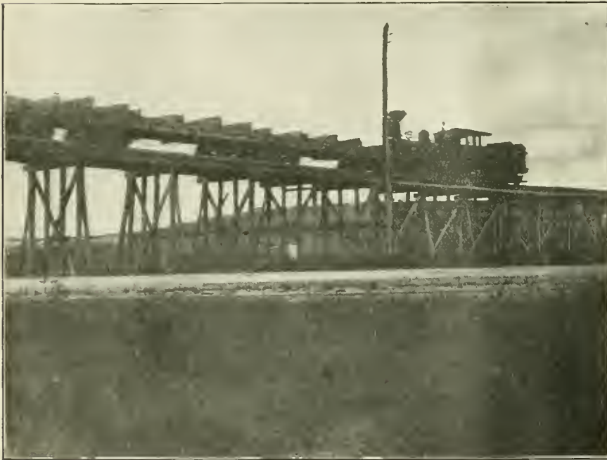
STANDARD GAGE RAILWAY CROSSING HIGHWAY BETWEEN QUARRY AND DAM—PART OF M'ARTHUR BROS.' PLANT.
